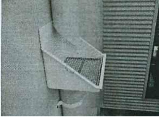
Figure 11: A typical mesh filter
