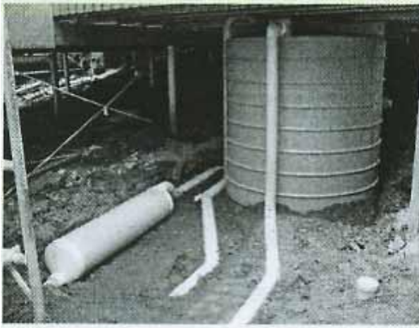
Figure 12: A typical first flush device
